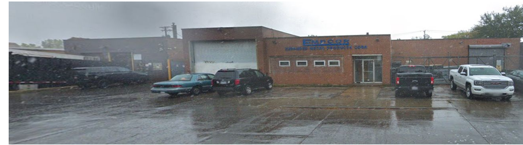
Figure 4. This is a steel manufacturing company in Archer Heights Neighborhood located in Chicago that uses heavy metals such as zinc.
